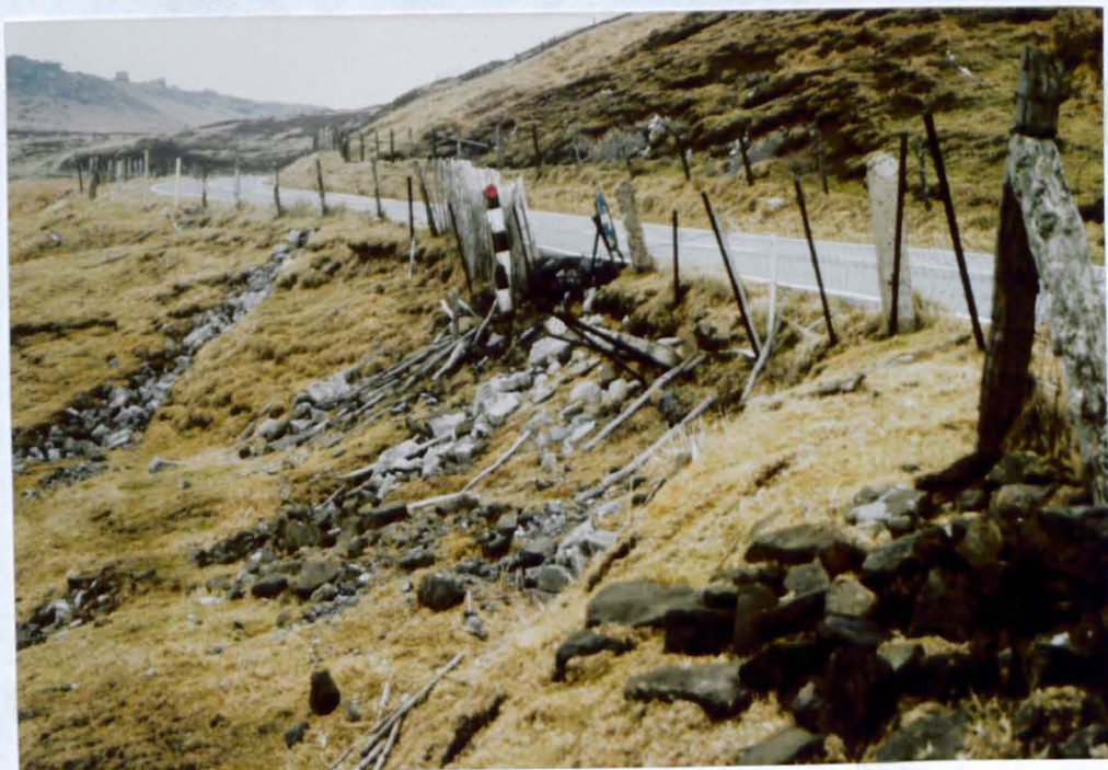
Plate 4. Landslide damage to a minor road passing below Higger Tor, Callow Bank.
