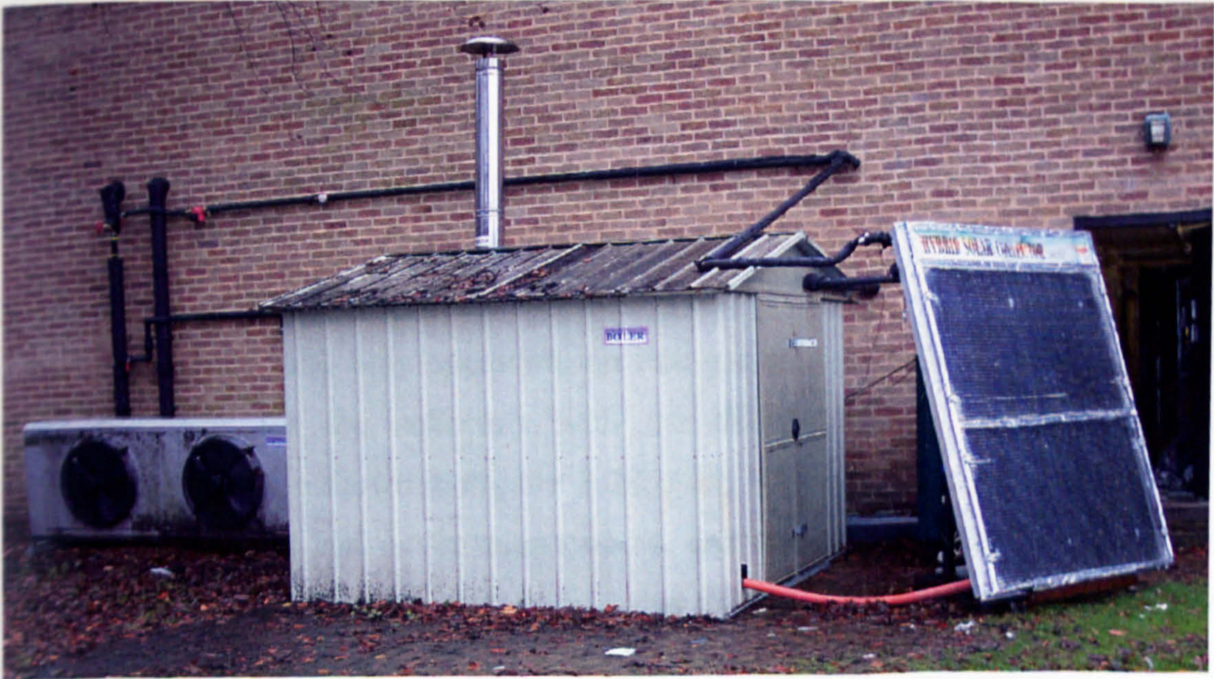
Figure 5-26. Layout of the integrated hybrid solar collector/CHP system – outdoor part
