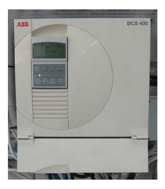
Figure 4.40: DC drive converter
