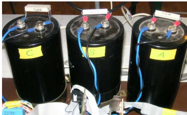
Fig. 5.16: Photograph of three-phase DC-link capacitors
